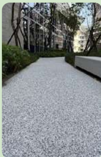
▲ Permeable flooring on the first floor to channel rainwater to the rainwater recycling tank in the basement.
